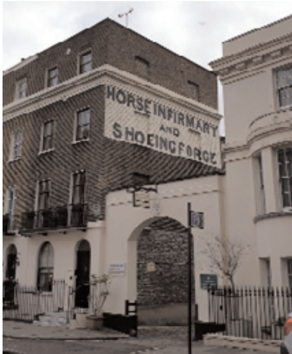
Right: Example of recently restored sign.
