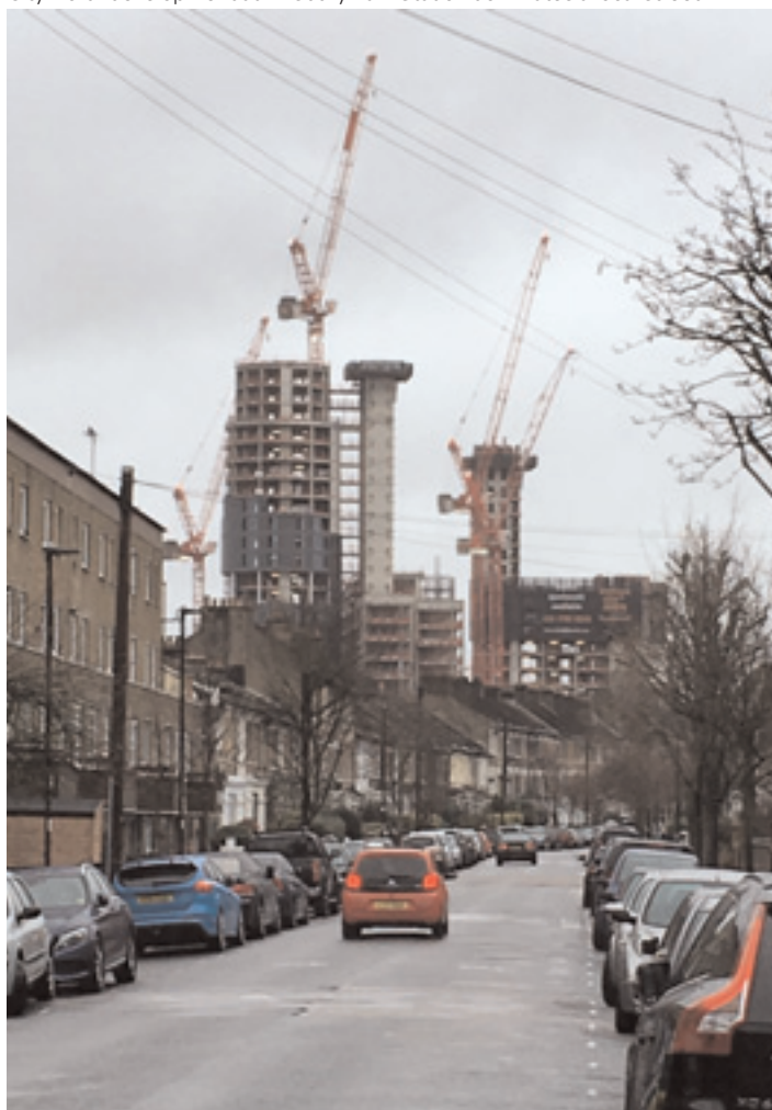
City North development at Finsbury Park Station dominates a local street
